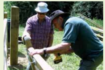
Volunteers constructing a new catching pen at Hutchinson's Bank
